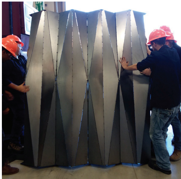
Fig. 7 Students in Flat Force Fold Form research studio preparing to move a 360lb a roof piece prior to installation.
